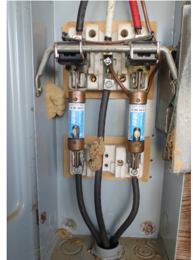
Photo 7: This generator battery is in serious need of cleaning and testing. Can you identify the problem? Photo 8: Each house disconnect will have a breaker or fuse to protect the wires and equipment on the load side. Inspect and clean all these fuses. Can you identify the problem?
