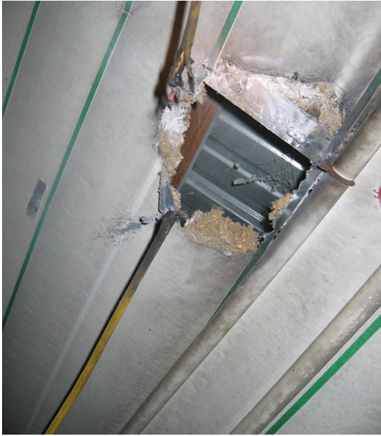
Photo 5: This grower allowed an inexperienced helper to install a new fan circuit and, as a result, nearly burned the building down. Thankfully, we noticed the flame and had access to a fire extinguisher. Photo 6: Not the best repair work we have seen, but the fan works now.
