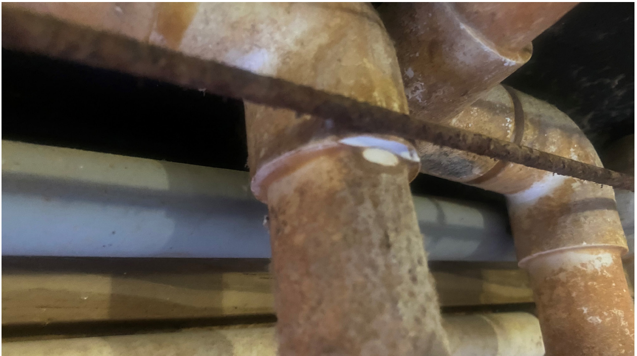
Photo 2: This is a similar picture showing the continuous steel rod rubbing directly into the 3/4-inch SCH 40 PVC water supply line in another house. Again, this is just a disaster waiting to happen and must be corrected ASAP.
